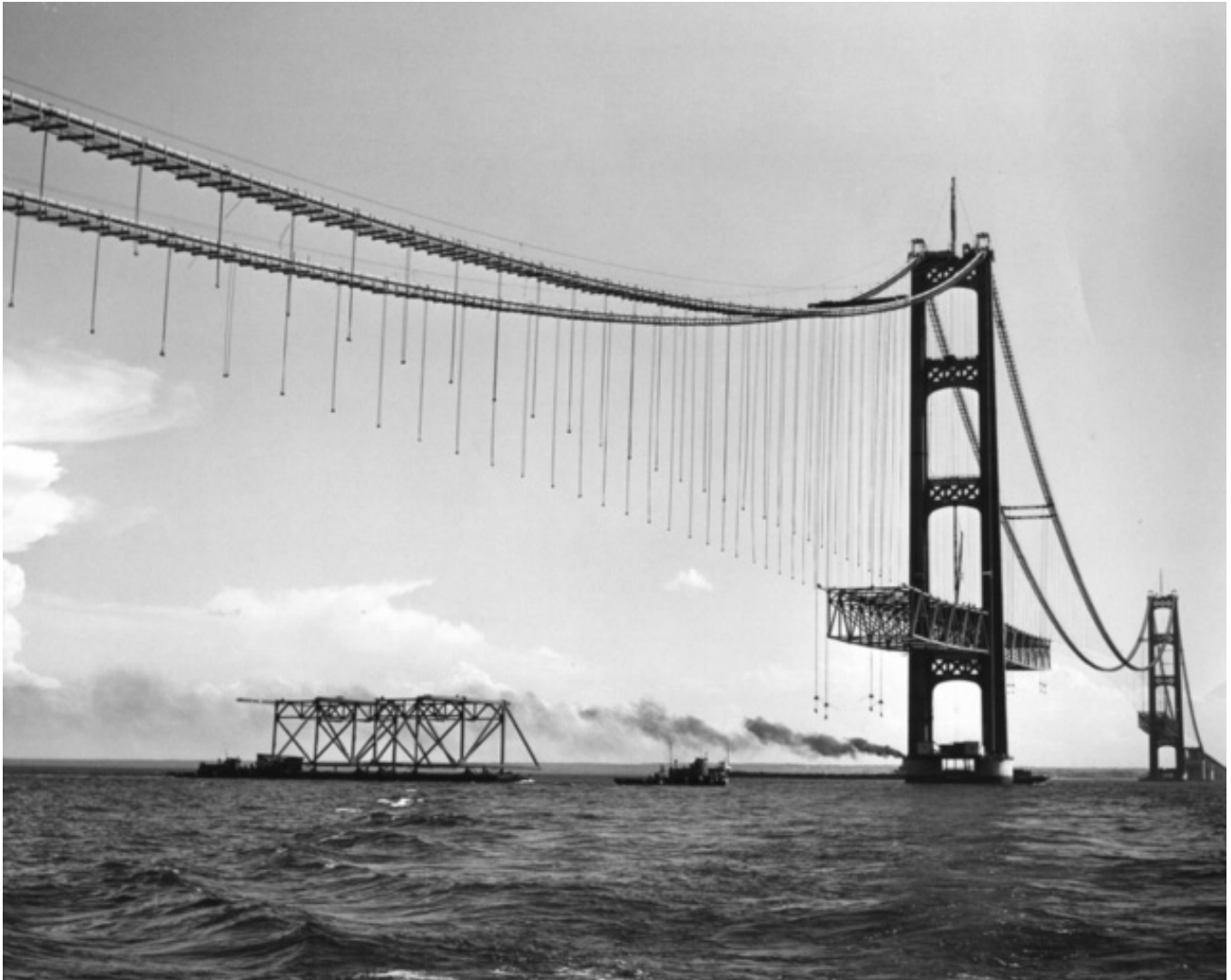
Truss Delivery by Barge. June 20, 1957. www.mackinacbridge.org/history/historical-construction-album/ . Accessed October 30, 2017.
